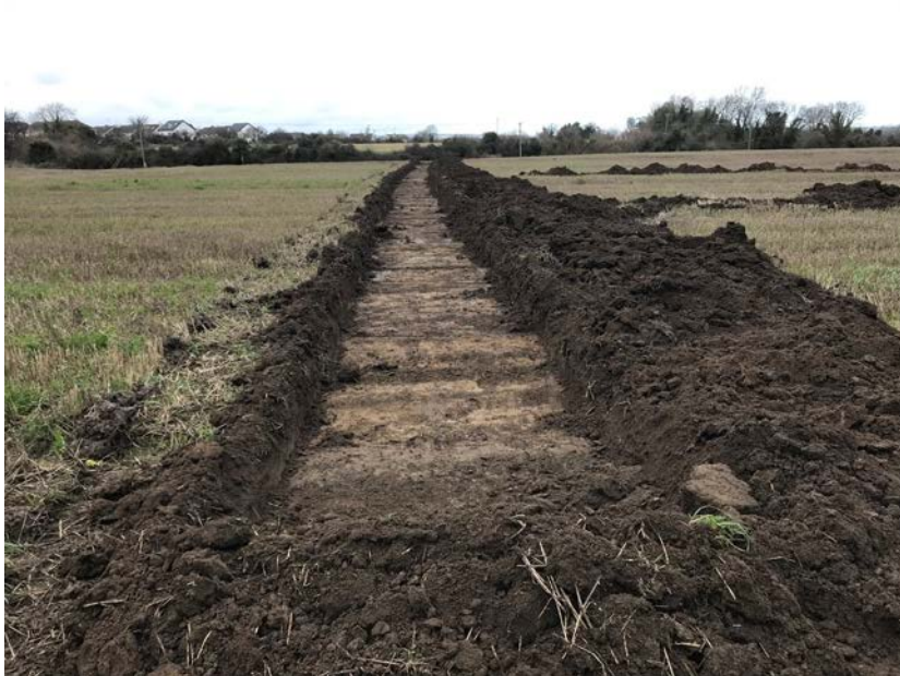
Plate 7: Trench 5, facing north
